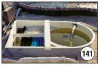
We recommend that all ponds be gravity fed from the bottom of the pond to a pre-filter settling chamber or a combination settling chamber/filter, before the water enters the main filter and pump. This system captures 85% of the solid waste and gives more time between cleaning of the main filter. The sump is easily cleaned with a dedicated trash pump in the bottom of the 60 degree chamber. We also manufacture both stand alone and combination settling chamber/filters.
