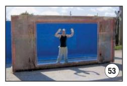
We can install large acrylic windows, up to 10' long x 6' high, on the side flat section of this tank in order to make an aquarium.
