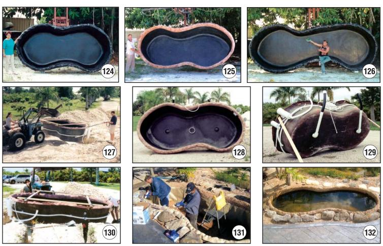
Our line includes three peanut shaped fish ponds. These ponds are 3' deep and have a smooth glossy gel-coat interior with a choice of several colors. The ponds have an undulating rock like textured flange around the top that can be painted or finished with adhesive and gravel to give a more natural look. These ponds are not free standing; they must be partially buried for proper installation. Extra heavy lay-up with foam coring is available if above ground installation is required.
